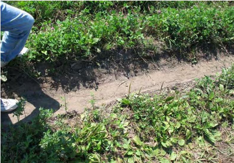
Photo 409, Point 4: Rutting on Levee Crest.
